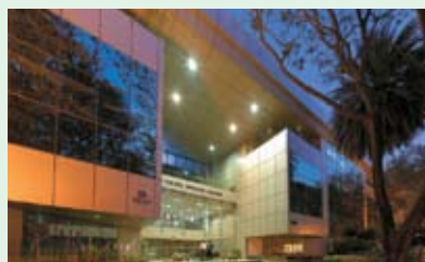
HULKUL BRIGADE CENTRE, THE CORPORATE OFFICE
